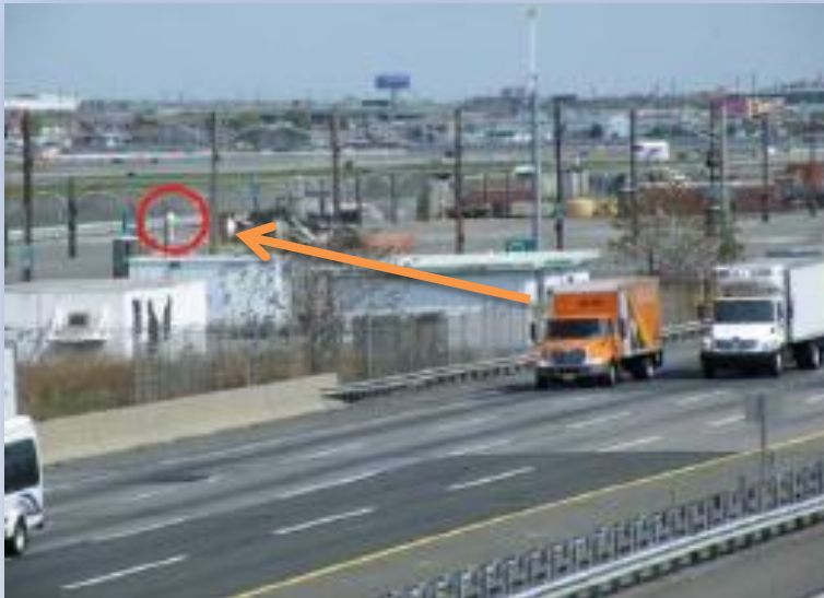
Impacted GPS Ground Antenna by Jammer
